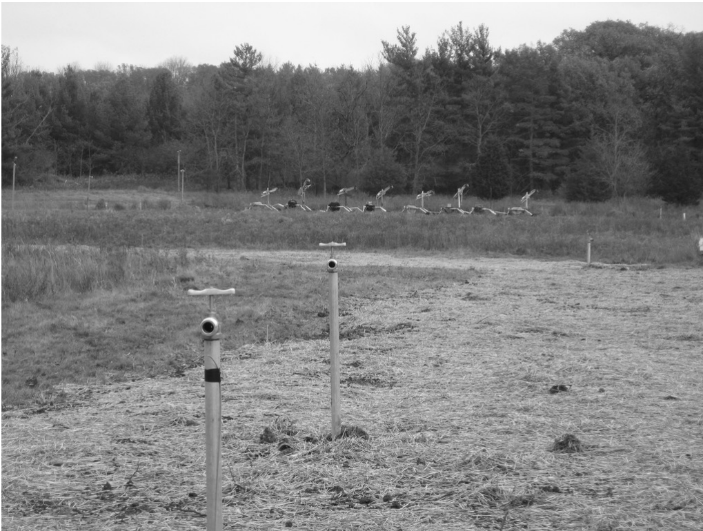
October 2010 In the foreground, are two of the new water hydrants installed this fall. In the background, snow guns await the advent of cold weather.
